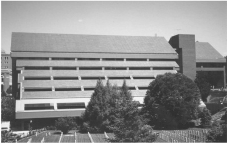
Figure 5.1 Roof-integrated photovoltaic system (Georgetown University in Washington, DC, built in 1984, 4,464 solar modules, 337 kW p total capacity)
